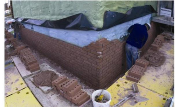
In typical installations, it allows workers to stand on the lower outrigger planks and to have material handy, on either the top outrigger planks or the platform deck. This concept will minimize risk of back injuries while providing a productive work area.
